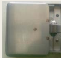
Align washer with flat plate
